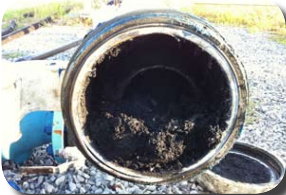
Pig Trap with Debris
