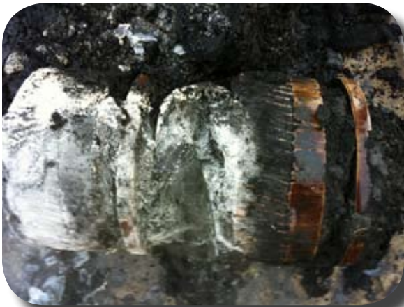
Dozer Pig with Debris
