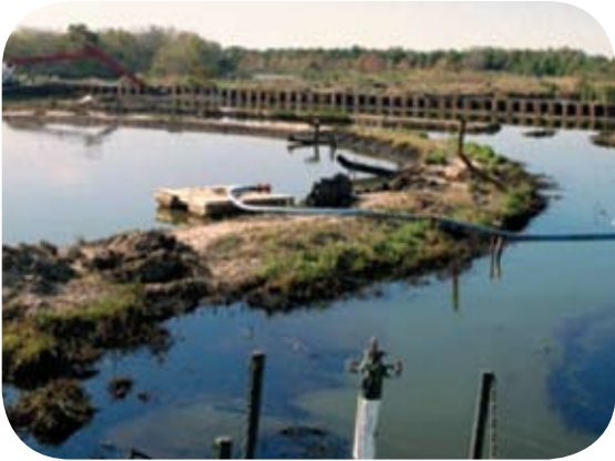
Produced Water Pit
