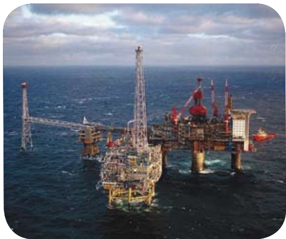
Statoil Sleipner 'A' platform
