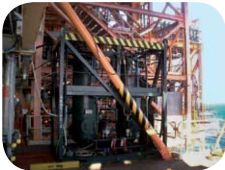
The CETCO RFV 3000 adsorption skid (below)
